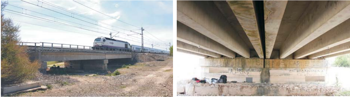
Figure 1: Old Guadiana river bridge.
