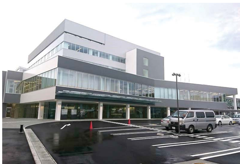
Figure 1: External appearance of the target building.
