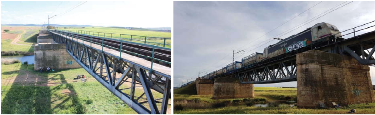
Figure 24: Bridge over Jabalón River (38°53'51.2"N 3°57'44.7"W).
