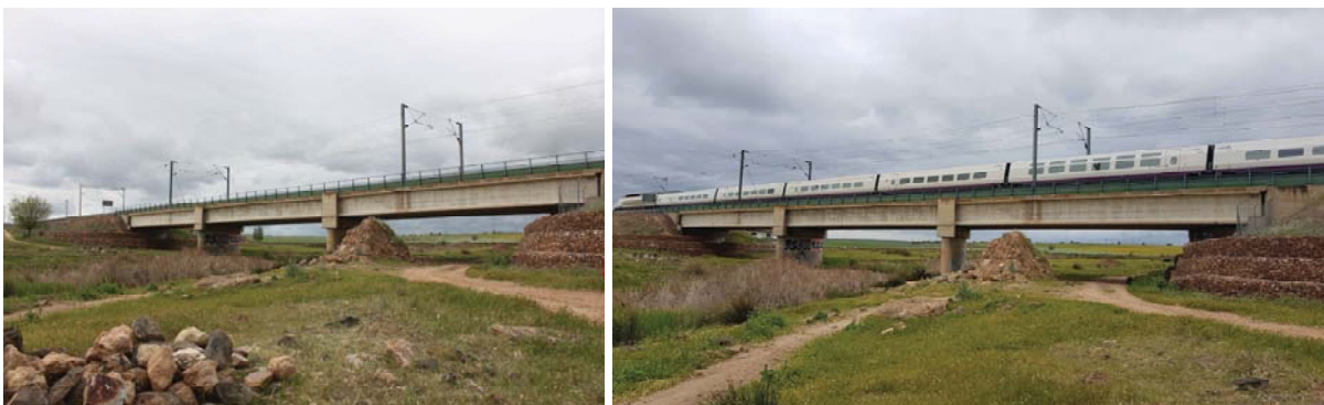
Figure 12: HSL bridge over Jabalón River ( 38^{\circ}53'51.3''\text{N} 3^{\circ}57'53.0''\text{W} ).
