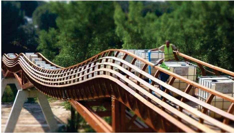
Figure 1. Loading test in a timber footbridge.
