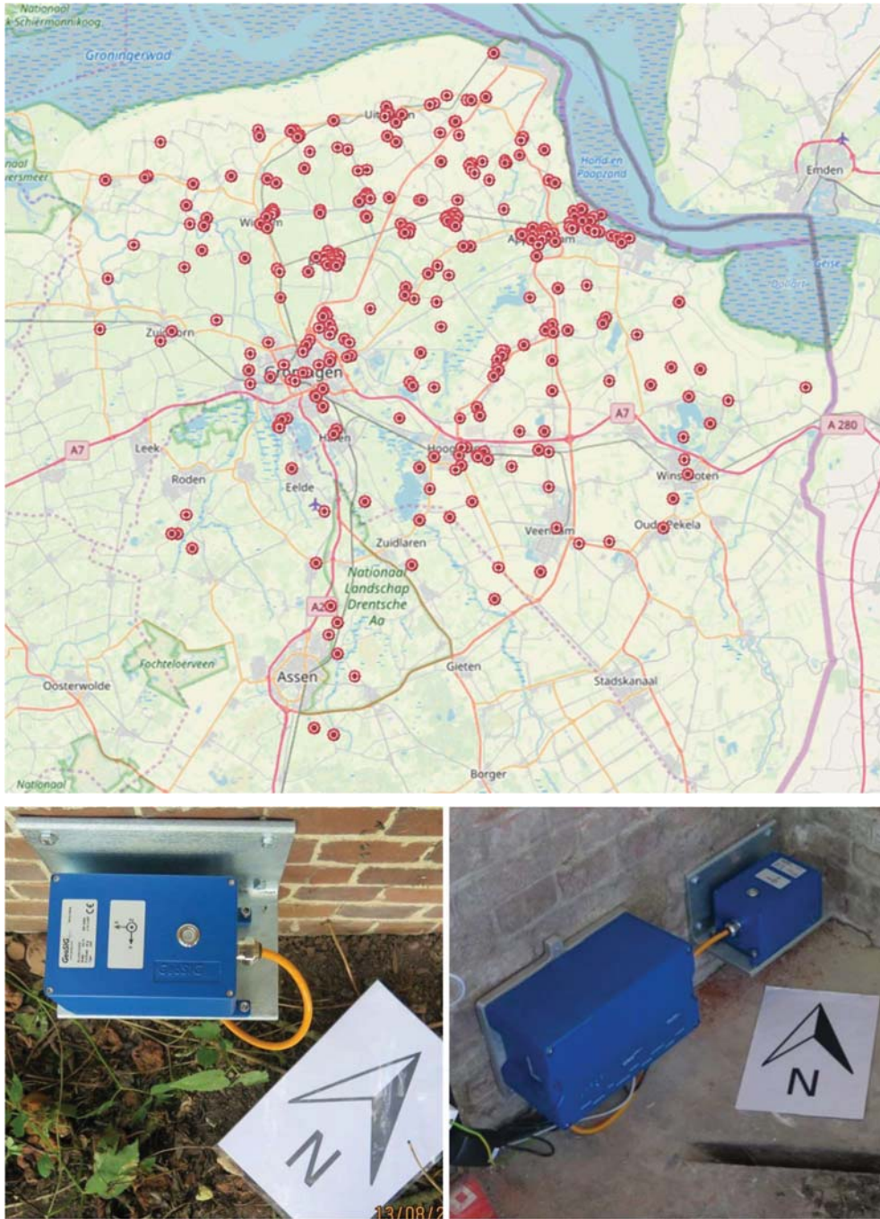
Figure 1: (top) Sensor locations in the building sensor network in Groningen, (bottom left) Geosig sensor near a stiff corner on the outside of a building, and (bottom right) a Geosig sensor near the stiff corner inside, the large box to the left is the recorder, the small box to the right is the sensor.
