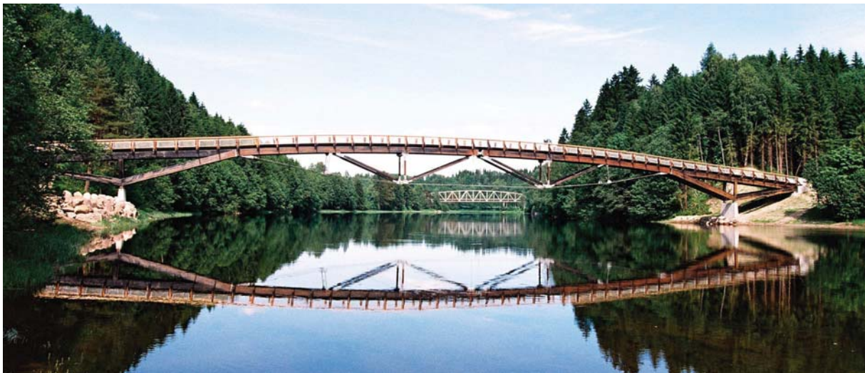
Figure 1: The Kjærra Bridge has a total span of 132m and a free span of 92m across the Numedalslågen River in Lardal, Norway. Photo: Lisbeth Michelsen
