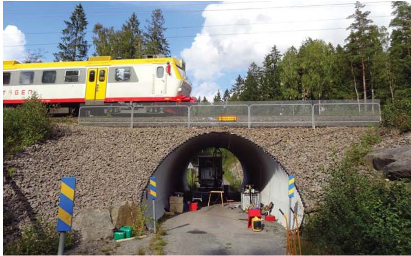
Figure 4: View of the Hårestorp bridge, during field tests in 2018. Passage of an X14 passenger train.
