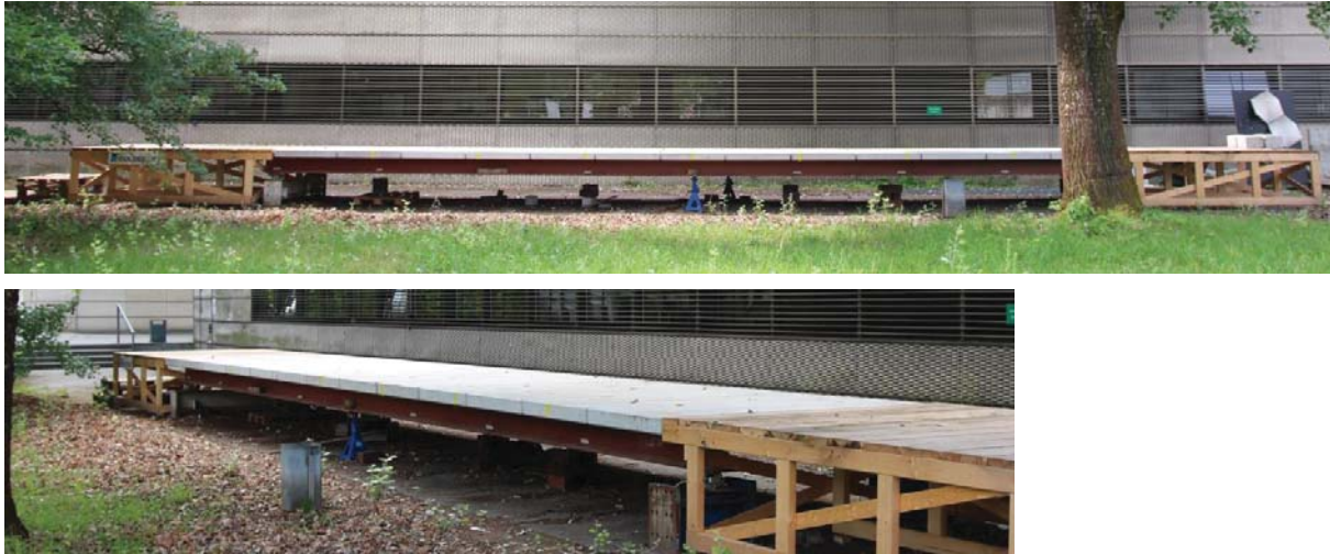
Figure 2: HUMVIB experimental pedestrian bridge (the middle support was removed during the experimental investigations)
