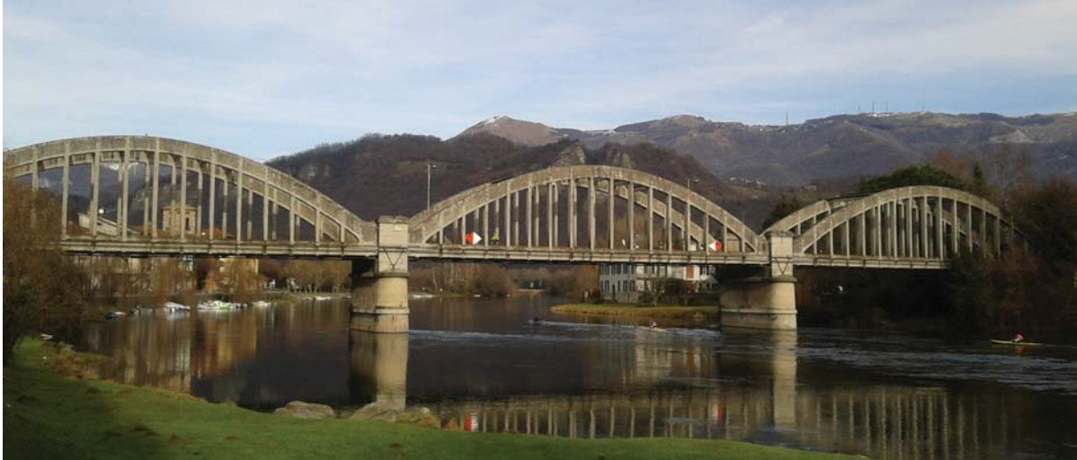
Figure 1: RC three-span arched Brivio bridge (1917) over the Adda river.
