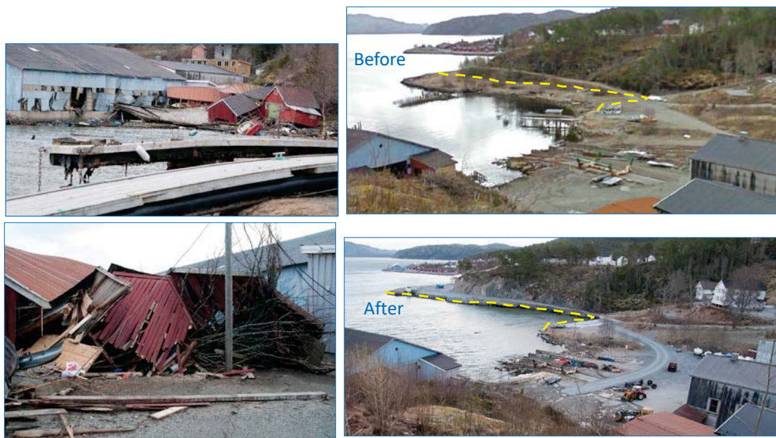
Figure 1 Photos showing damage caused by the Statland landslide. The right hand side photos compare the situation before and after the landslide with yellow dashed line showing the shoreline after the slide.
