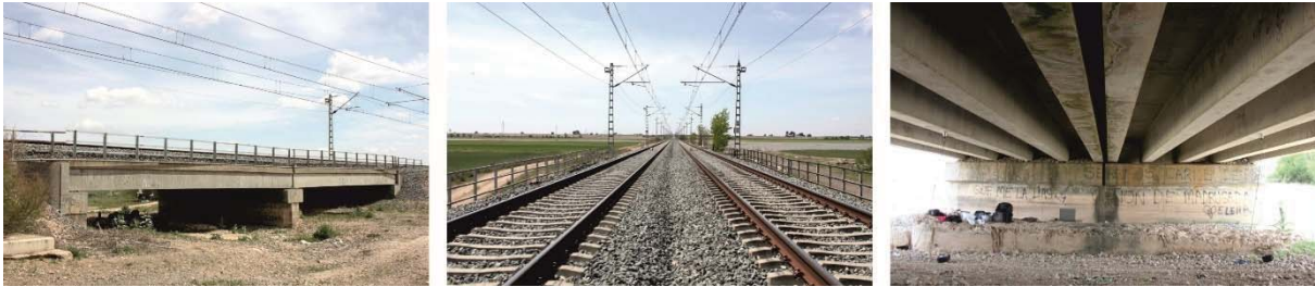
Figure 1: Old Guadiana Bridge photographs.
